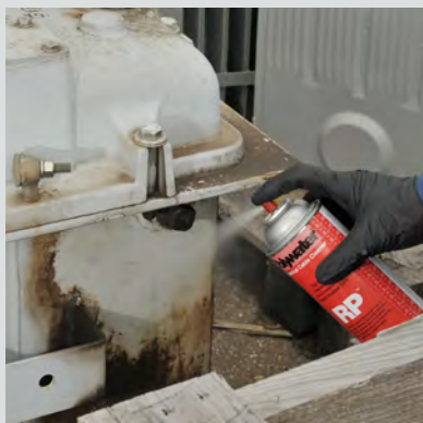
Removing transformer oil residue
