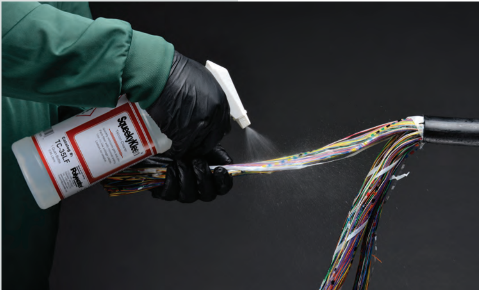
TC-35LR cleaning 200-pair copper cable
