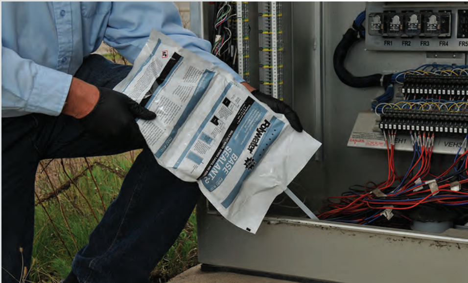
Polywater PedFloor burst pack installation
