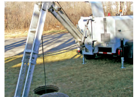
Large cable pulling machine
