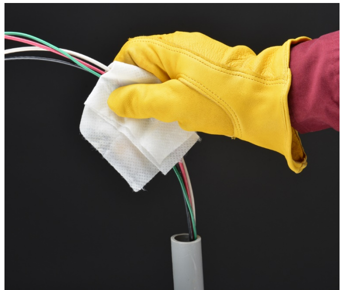
Wipe application with Polywater SPY-D20
