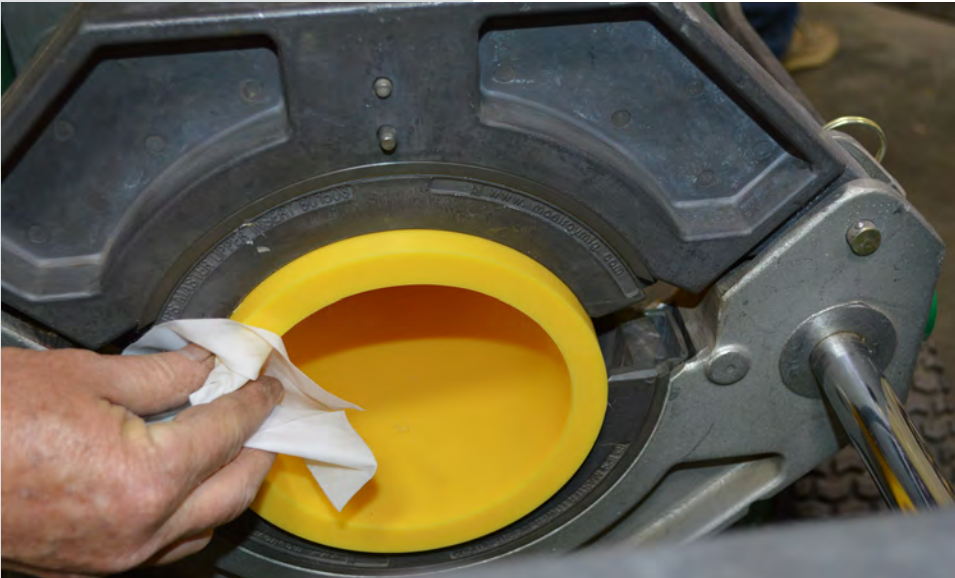
Cleaning after cutting PE gas pipe
