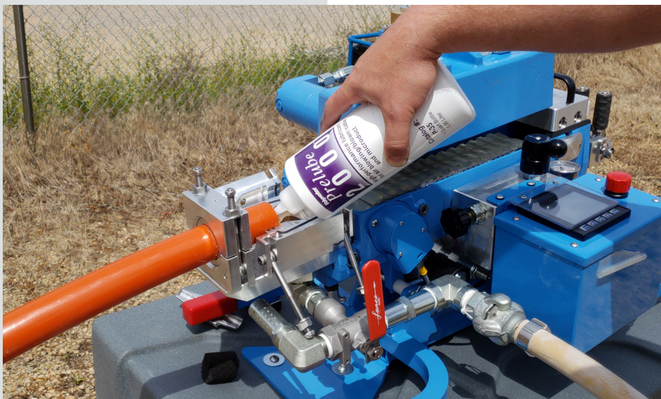
Prelubricating conduit prior to blowing fiber optic
