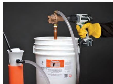
F applied to duct with an LP-D5 pump
