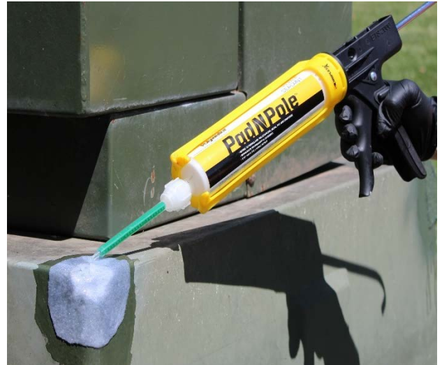
Fabric saturated with the high-strength, two-part resin creates a permanent Pad N Pole Repair.
