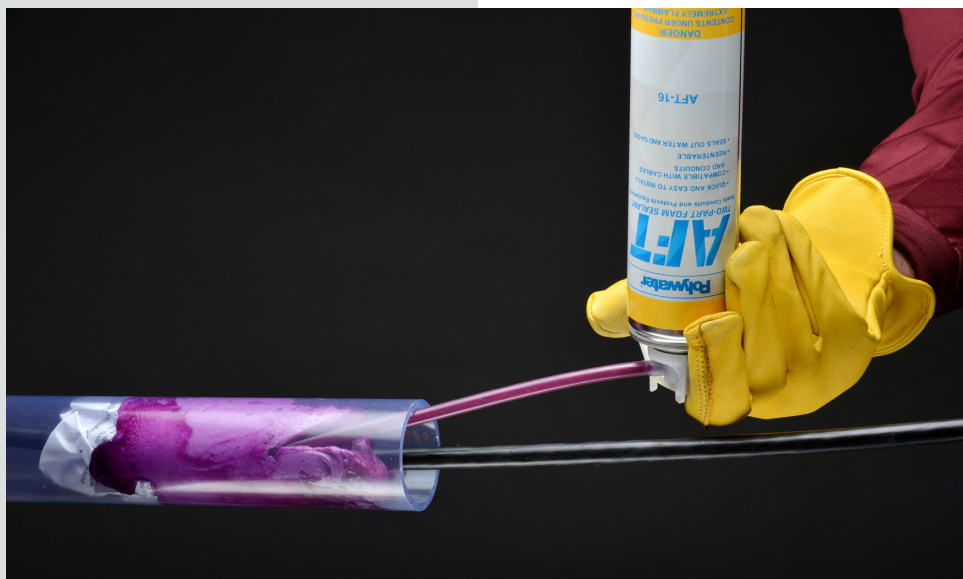
Installation of Polywater AFT-16
