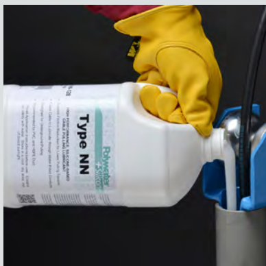
Pouring lube into a conduit stub-up
