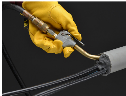
Blowing CableFree through conduits
