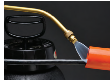
FTTx applied to duct with a sprayer pump
