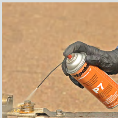
Loosening pole line bolts
