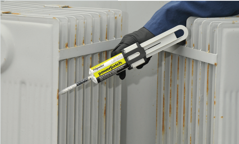
Transformer radiator fin repair
