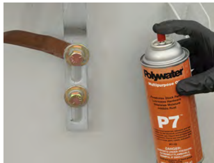
Liberally apply P7 to loosen
