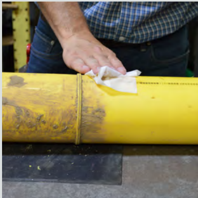
Removing dirt with the EFW-1
