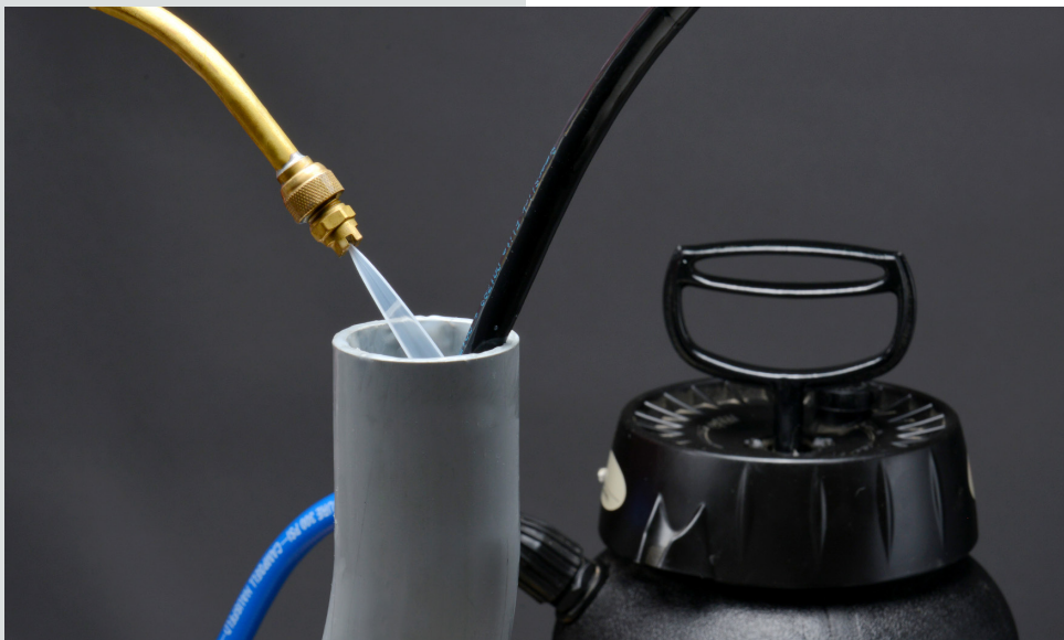
Spraying SPY lubricant into a stub-up
