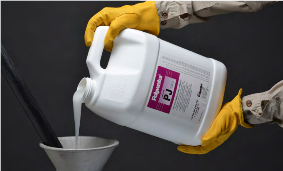
Polywater PJ being poured into a feeder tube
