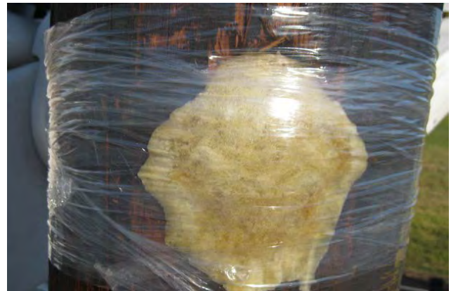
Woodpecker damage repaired with UPR™ Pole Repair
