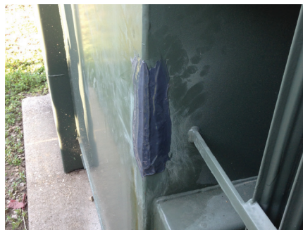
Pad-mounted transformer repair
