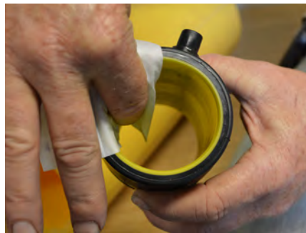
Cleaning fitting prior to fusion
