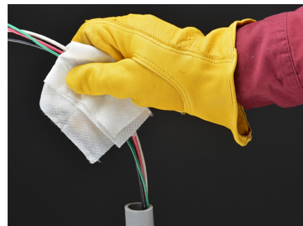
Using presaturated SPY lube wipes
